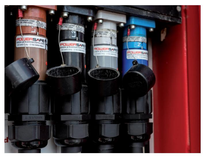
With increased demand for temporary high-power systems in entertainment & industrial applications, the choice of high current connectors is critical to ensure safety and reliability for every use. Designed to connect single & three phase high current power circuits, Powersafe single pole connectors are at the forefront of both safety and technical capability.
